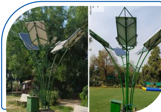
Glimpse of UPNEDA Solar Tree Project
